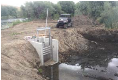
Benton County Voluntary Stewardship Program funding was used to install water control structures at Mast Farms to increase floodplain functionality. Photo by Bob Montgomery, Anchor QEA
